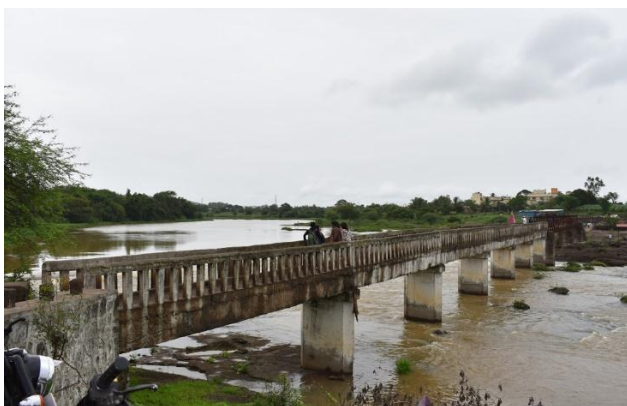
Fig.1 Kund-Mala Bridge near Talegaon over Indrayani River
