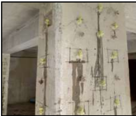
Fig -1: Epoxy Grouting on Column
