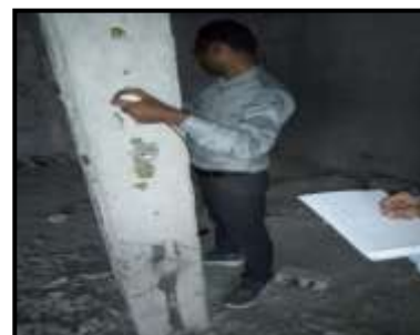
Fig -6: Ultrasonic Testing on Column
