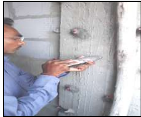
Fig -2: Micro Fine Cement Grouting on Column
