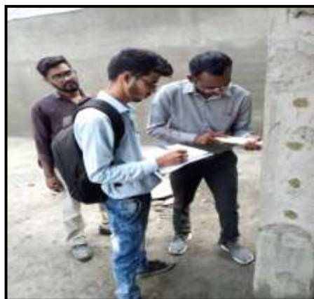
Fig -4: Rebound Hammer Test on Column
