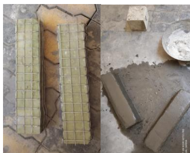
Fig 9: Retrofitting of beams
