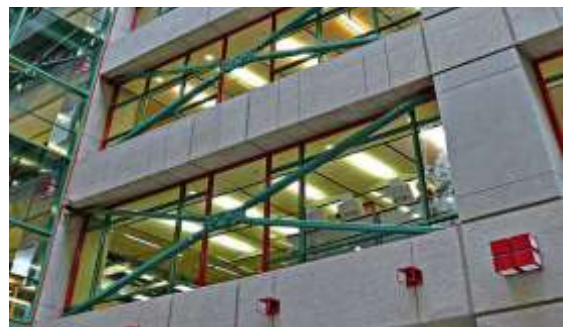
Fig - 1: Concordia's Library Building Connected with Pall Friction Damper
