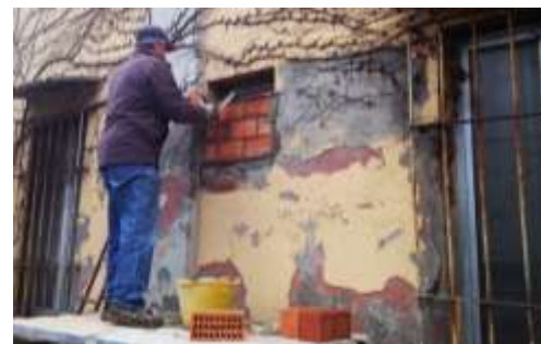
Figure -2: Walling of fenestration of Torrione Fodesta [4]
