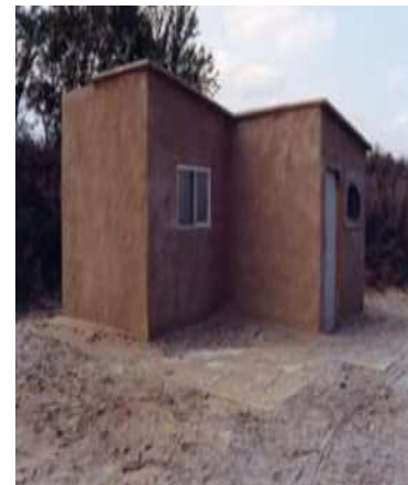
Fig -3: Finished grancrete building
