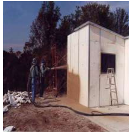
Fig -2: Spraying of grancrete mortar
