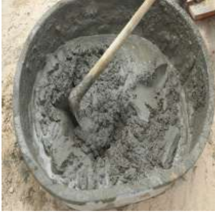
Fig -9: Mixing of mortar
