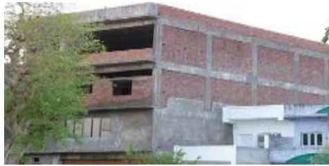
Fig. 2- RC frames with masonry infill walls
