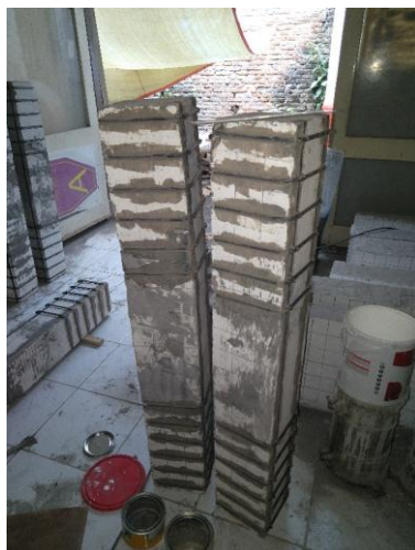
Fig -6: Beams after retrofit with external steel confinement Ø6-60
