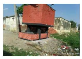
The upper wall which will be covering the 5000ltr tank has a height of 6.6fts and has the corners of 9 inches and the walls of 4 inches. The brick used in this wall is also 1<sup>st</sup> class brick. The ratio of sand and cement is same as of the lower wall.
