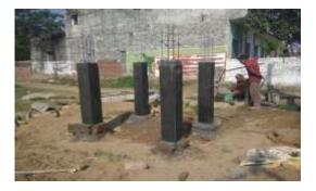
The dimensions of the column are 9x 9 inches and the height of the column above ground surface is 48 inches and below the ground is 16 inches.
