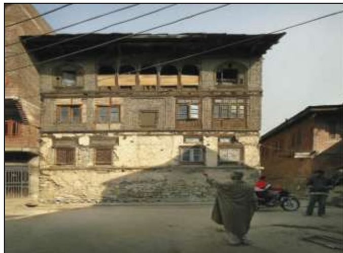
Fig 4 : Showing Taq construction in Srinagar (Symmetrical layout of windows is characteristic of taq and hence this name) (Source: 'Randolph Lagenbach book-Do not tear it down).
