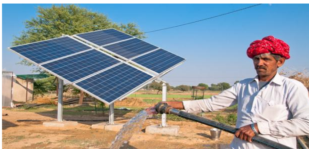
Figure1.3 Solar Power Plant for Farmer
