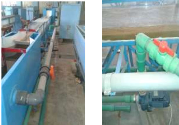
Figure (7) the pipes, the valves and the pumps.
