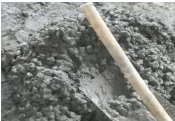
Fig.3 Mixing of the materials
