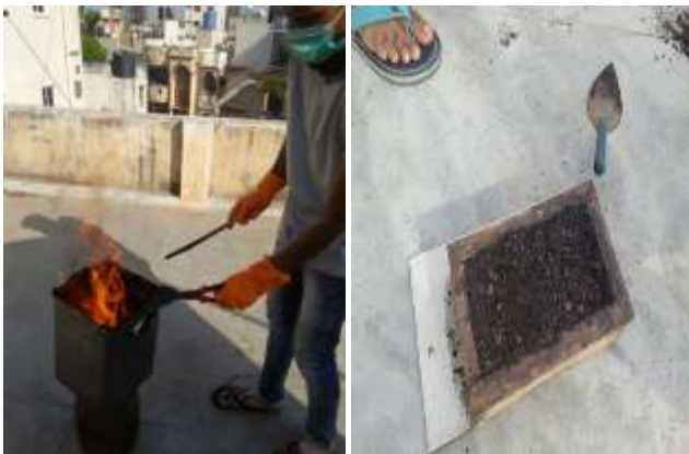
Fig -2: Plastic Paver blocks preparation
