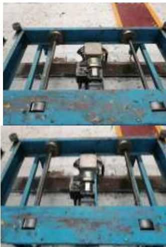
Fig -5: Cleaning of Roller bed
