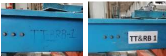
Fig -6: Roller bed Tag replacement at WBS
