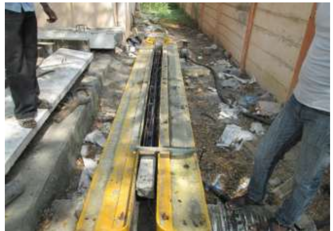
Fig.1 Steel reinforcement placed in the mould
