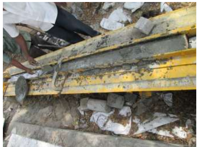
Fig 2 Casting of Reinforced concrete beam in the laboratory
