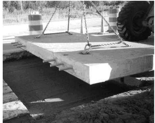
Figure-3. Installation of panels by Michigan method (Olidis et al. 2010)
