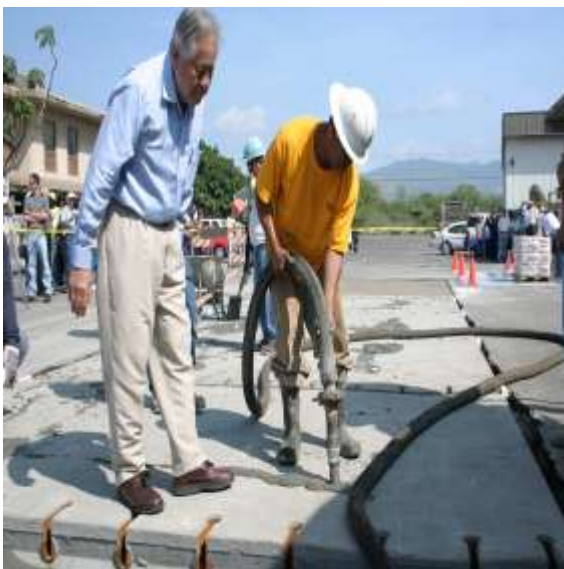
Figure.2 Grouting within Kwik slab panels (www.kwiklab.com 2011)
