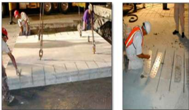
Figure-5. Uretek Fiberglass Tie Installation Process (Olidis et al. 2010)
