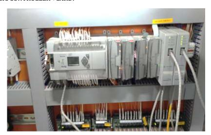
A PLC has a focal preparing unit (CPU) that can oblige an application program and info/yield modules. Plant and hardware controls and procedures are executed by guidelines put away in a PLC memory. The PLC memory stores the estimations of clocks, transfers, sequencers, and counters. The PLC offers certain focal points, for example, dependability, minimal effort, and can be re-customized.
