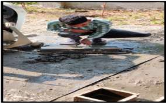
Fig -6 Beam Casting
