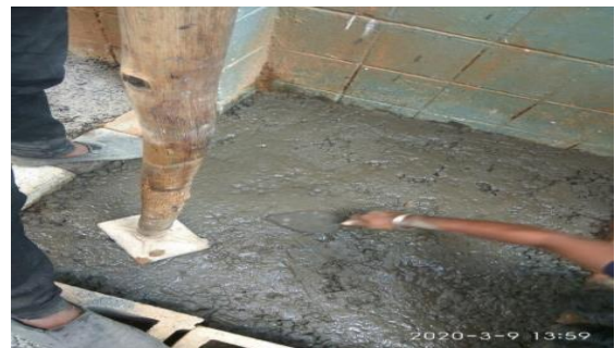
Fig - 8 : Laying of Concrete containing Fly Ash and Activated Carbon
