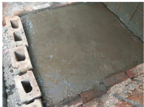
Fig - 10 : Finishing of Self Repair Road
