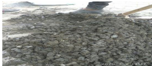
Fig - 9 : Laying of Fiber Reinforcement on Top Layer
