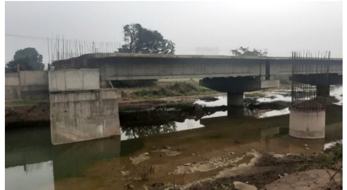
Fig -1: Quality of bridge work
