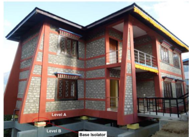
Fig-5: Prototype base-isolated masonry building located in Tawang, India
