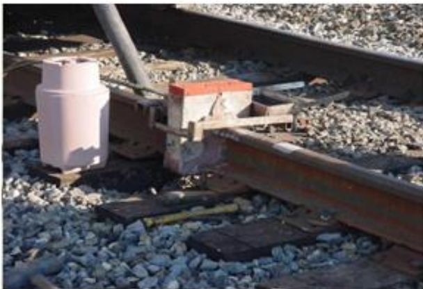
Fig 4: Installation of mould and crucible
