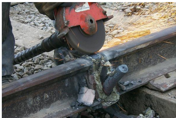
Fig 6: Post-weld finishing
