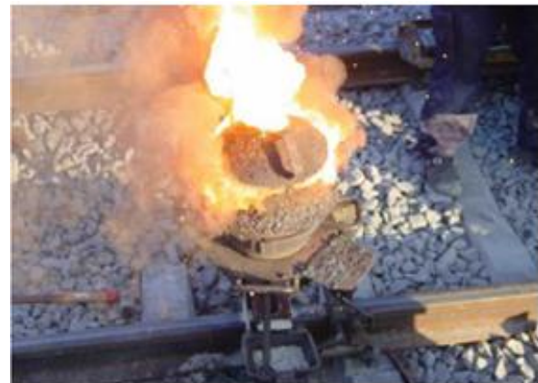
Fig 5: Thermite reaction in Crucible
