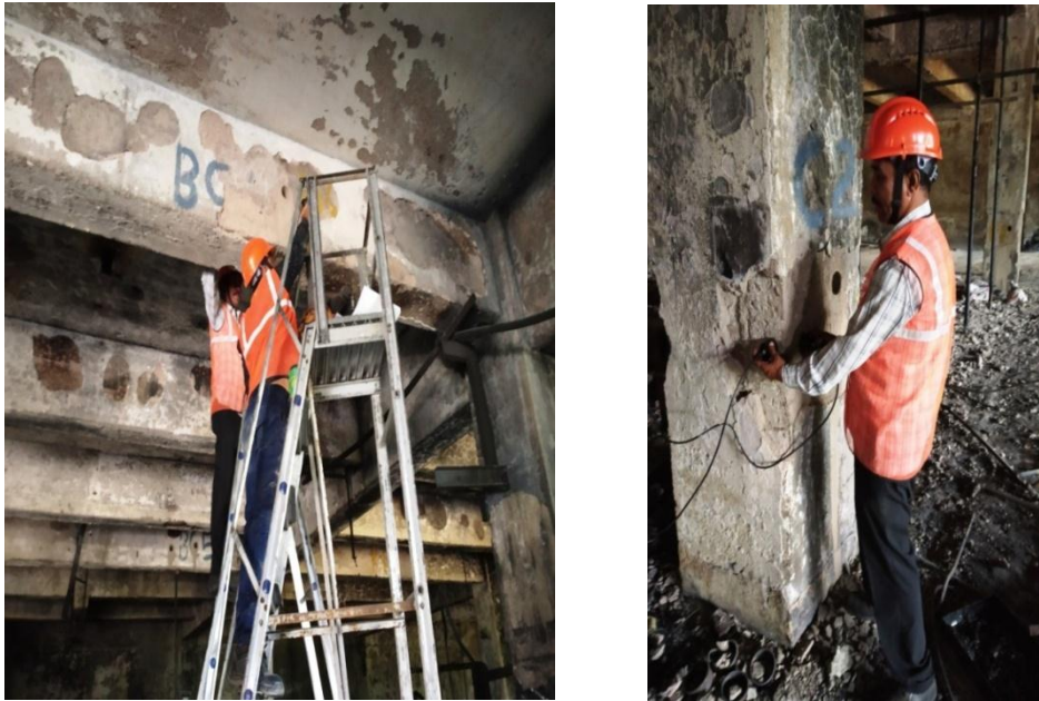
Figure 2: USPV test on column and Beam
