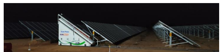
Fig.8: Implementation on Solar plant
