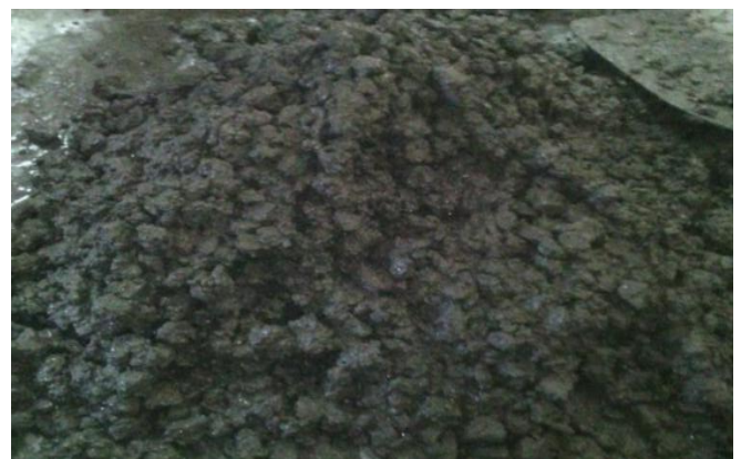
Fig-2: Mixing of Concrete
