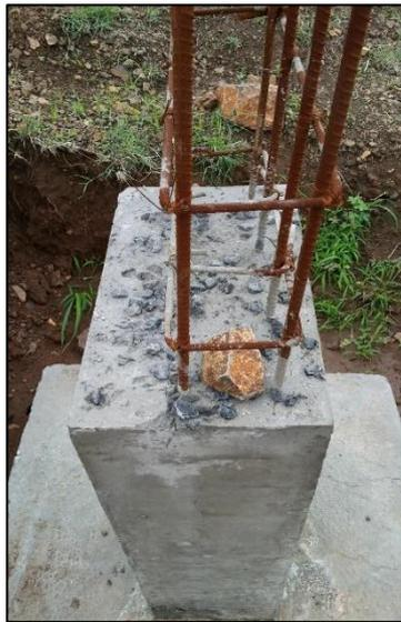
Fig.- 3 Improper Covering
