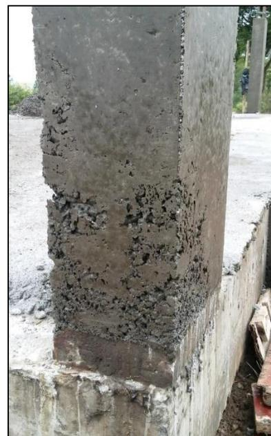
Fig.-2 Commonly Found Defect - Honeycombing
