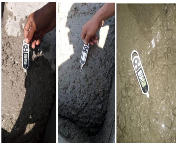
Photos of fresh concrete Temperature.
