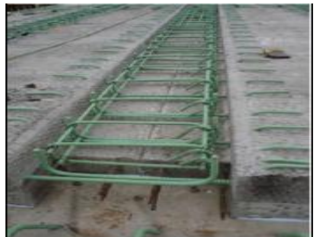
Fig -1: ABC Closure Joint
