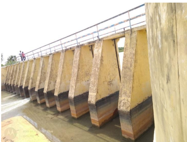
Figure -23: Check Dam
