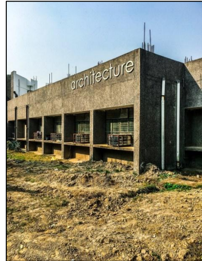
Figure 1: Department of architecture, A.M.U
