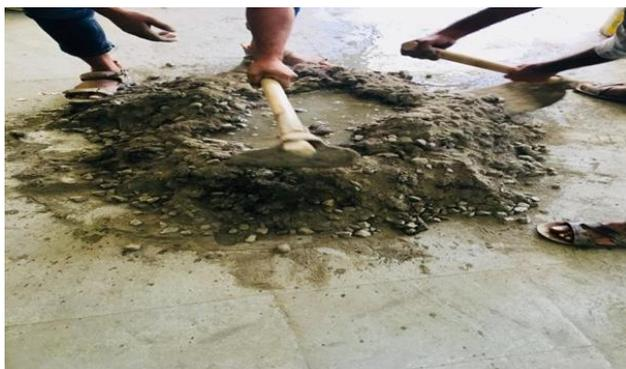
**Figure-2 Hand mixing of Concrete**
