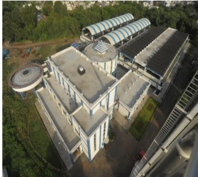
Fig:-Figure show water recycling plant
