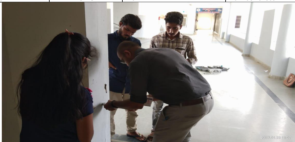
Fig 3.2 Conducting rebound hammer test
