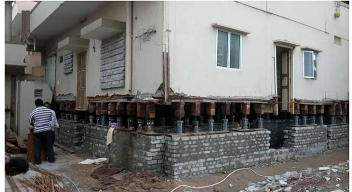
Fig. 1. Elevating house using Jacking Technology.
