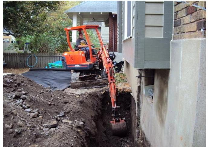
Fig. 4. Excavation around foundation.
