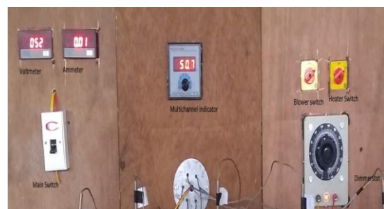
Fig -4: Control Panel
