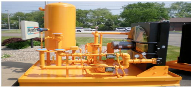
Fig 1.2 Closed-loop Dry Cooling Systems
