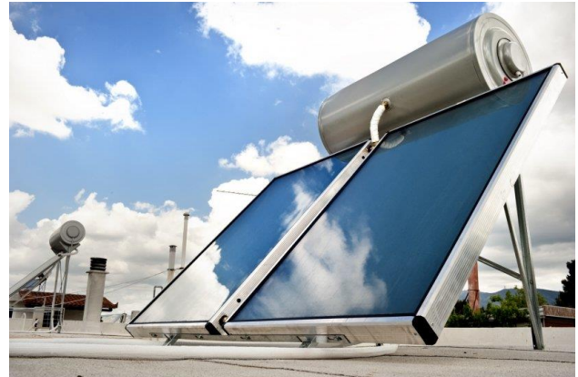
Figure 3: Passive solar water heater
