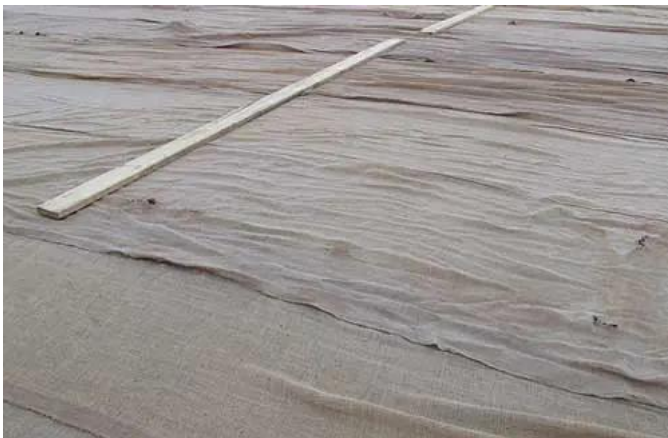
Fig -5: Wet Membrane Covering concrete curing mechanism (Structural Guide 2021)
