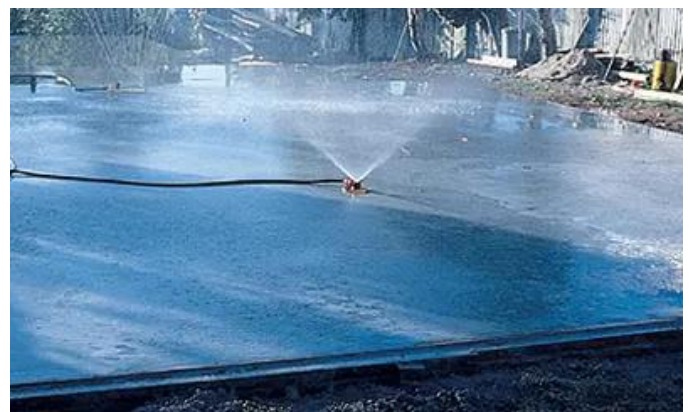
Fig - 4: Water Sprinkling concrete curing mechanism (Structural Guide 2021)
