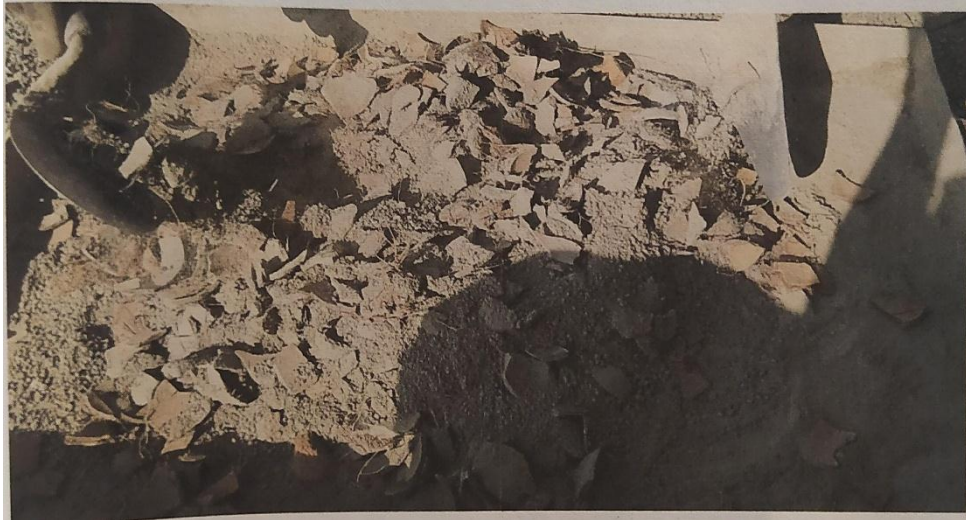
Fig: mixing of materials
