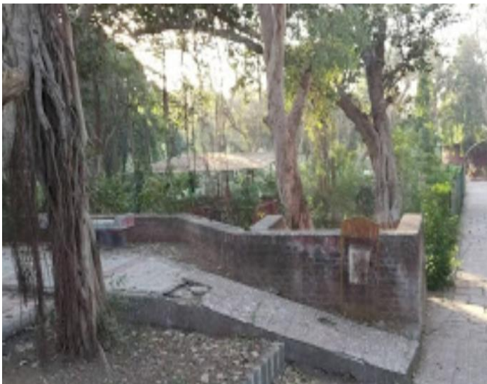
Fig-2 Inaccessible ramp facility at Jawaharlal Nehru garden
