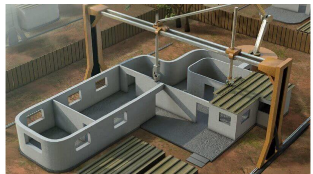
Fig.1. Working of 3D Structural Printer
