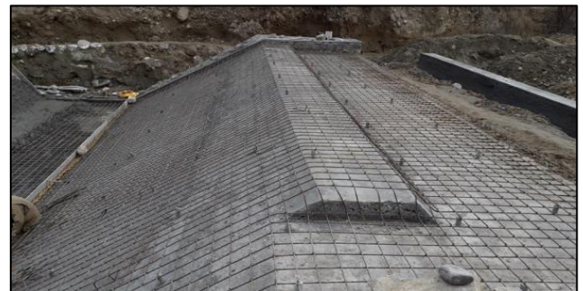
Figure 7: Headworks under construction:
