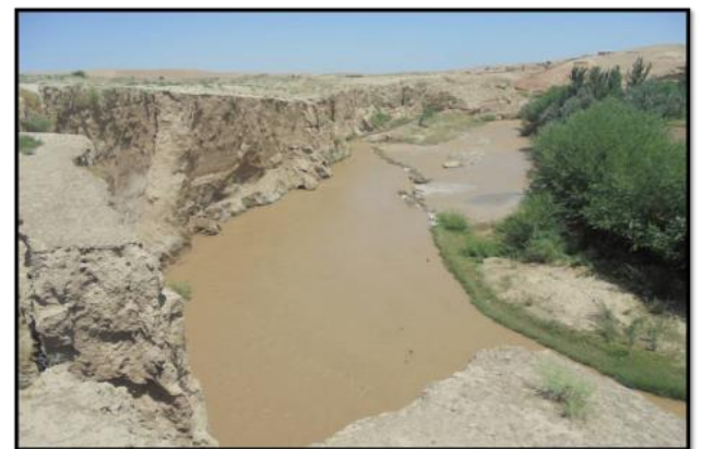
Figure 5: Present condition of main canals
