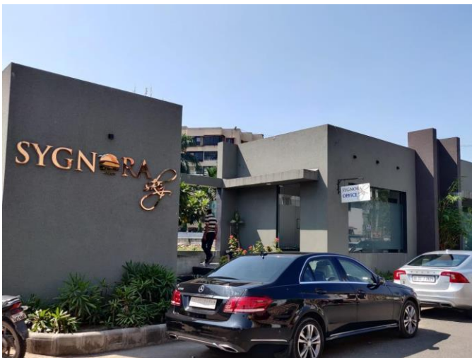
Fig-6 Sygnora Sky Residential Building
