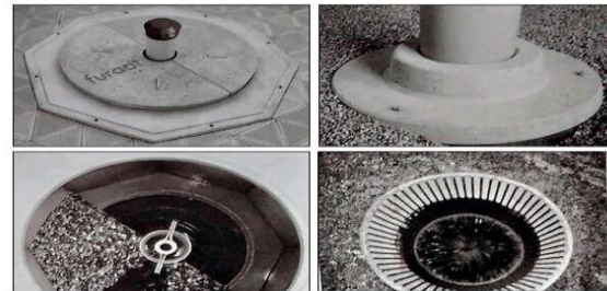
Fig 4.3: SFM recharge pit top view
