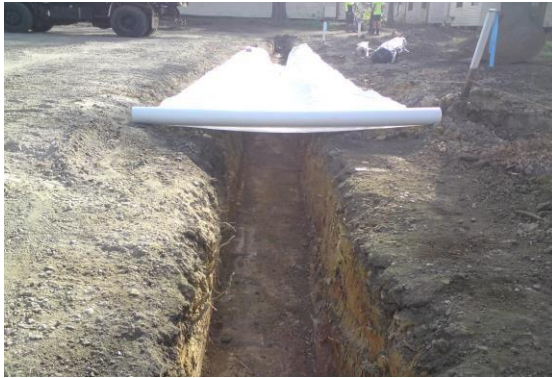
LAYING GEOTEXTILE
