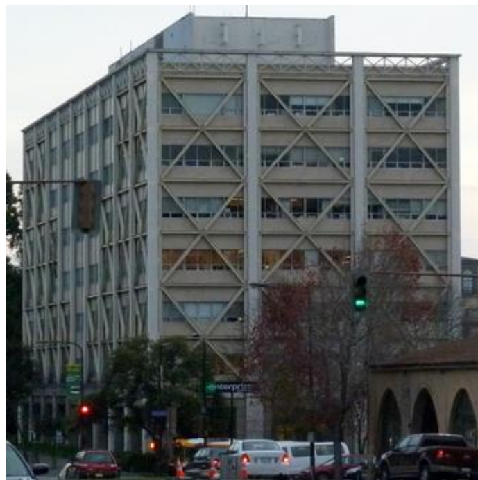
Figure 0:4 Braced Frame System
