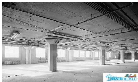
Fig -1: Flat Slab
