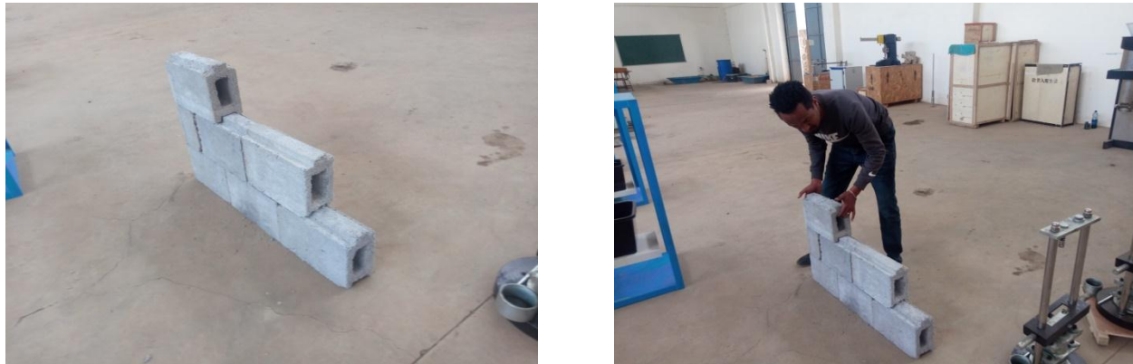
Figure 6: Coursing a masonry using IHCB (Mortar - less) units
