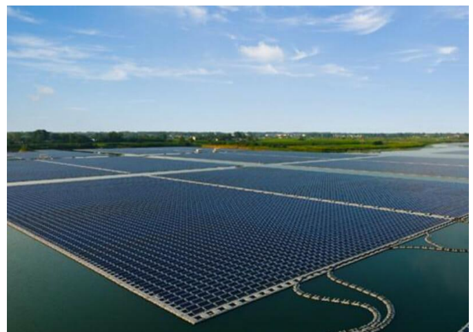
Fig -1: floating solar plant of 25MW on omkareshwar reservoir in Madhya Pradesh.
